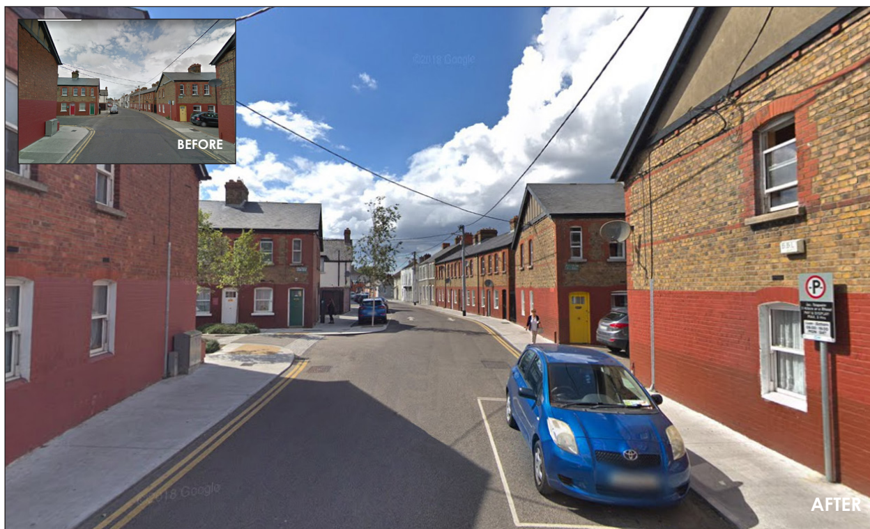
View towards junction of Cross Avenue and Wolf Tone Avenue. Works include tightening of corner radii (new kerb line/footpath widening and build out), entry treatment and use of on-street parking to create a horizontal deflection (image source Google Street View).
