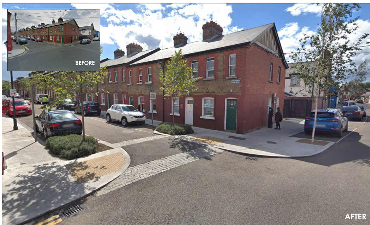
View from Cross Avenue to Desmontf Avenue. Works include tightening of corner radii (new kerb line/footpath widening and build out), entry treatment, street tree planting (including plated tree pits)(image source Google Street View).
